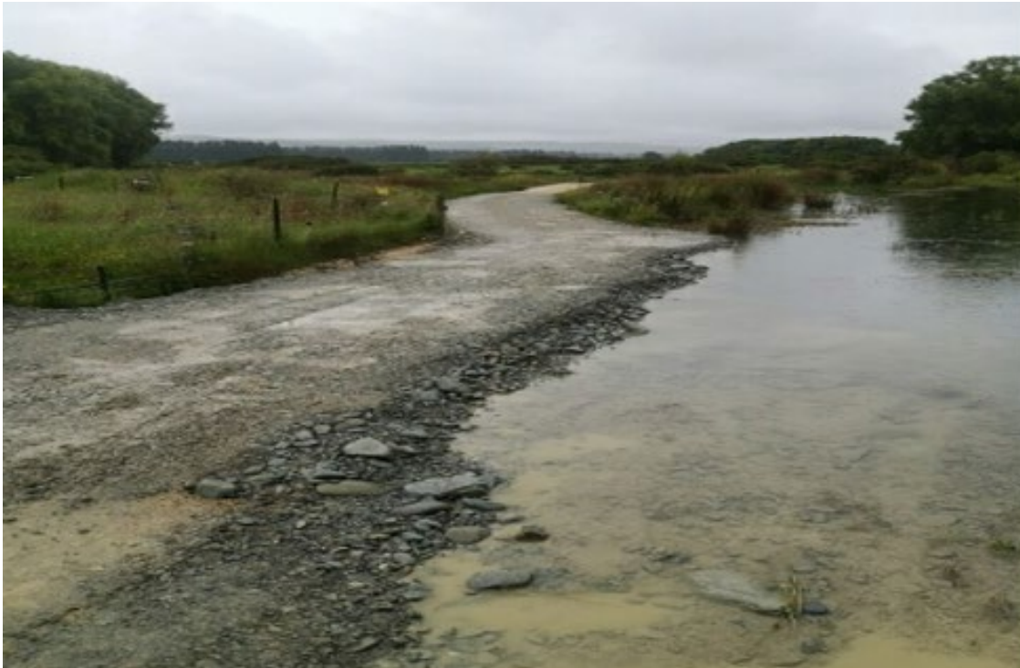
Figure 8 Raised Track near Otiake River
