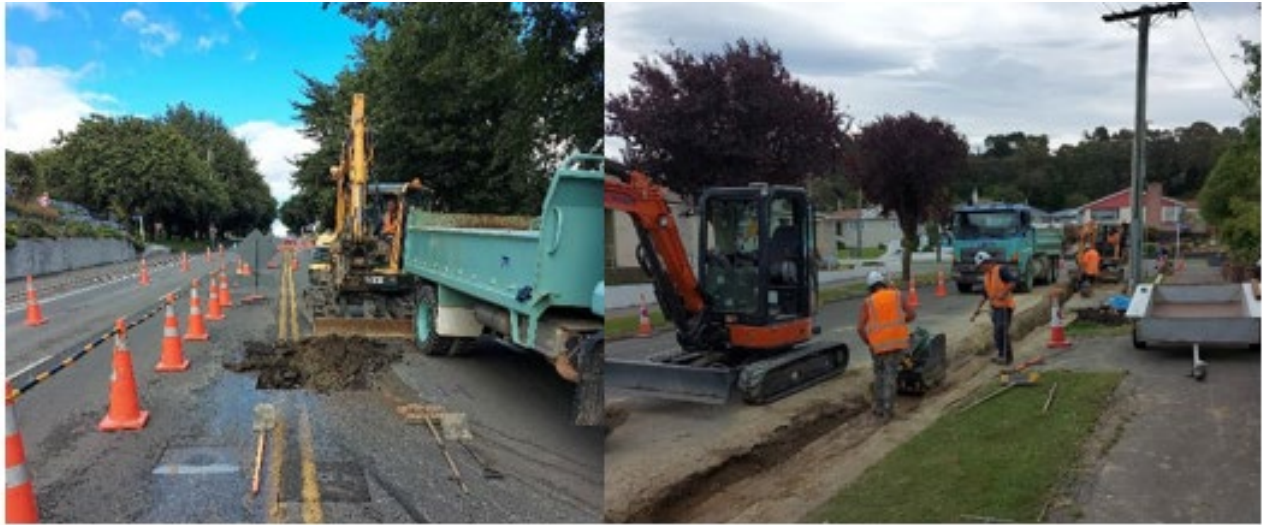
Figures 1 & 2 Ōamaru watermain installation
