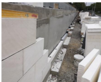
Oamaru Stone facing in progress.
