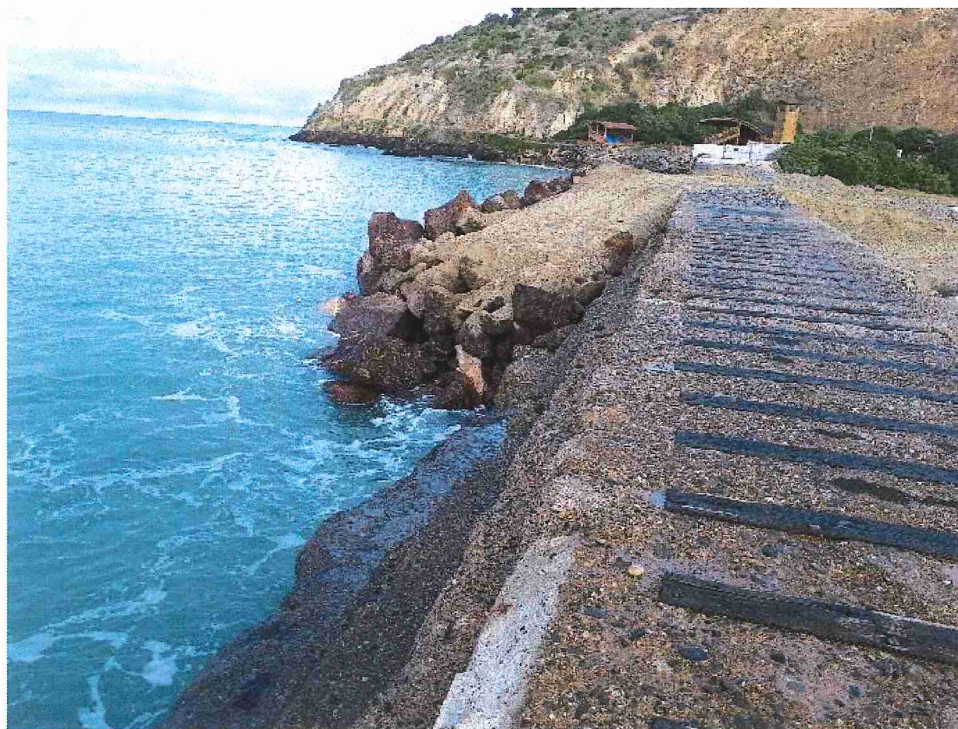
Breakwater rock armouring looking south towards penguin colony
