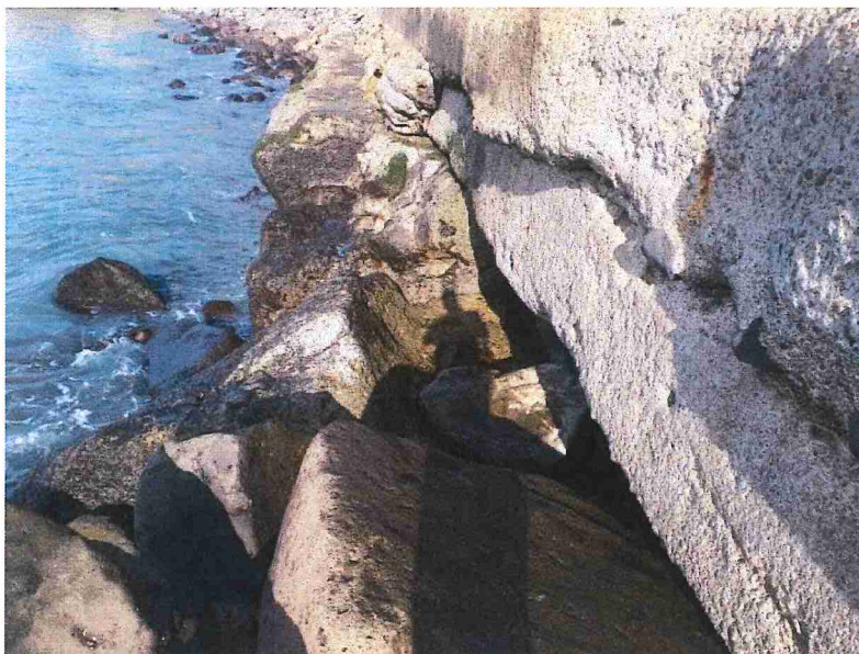
Photograph of breakwater showing concrete deterioration, prior to the latest rock armouring campaign
