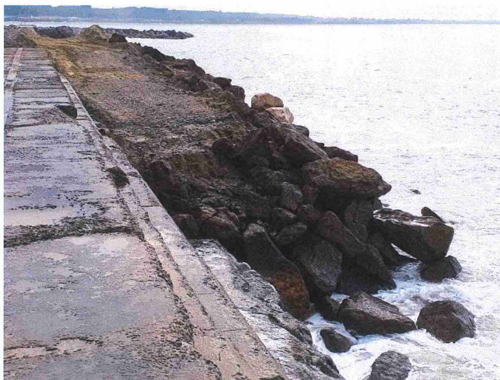
Breakwater rock armouring looking north towards Ramsay's Extension
